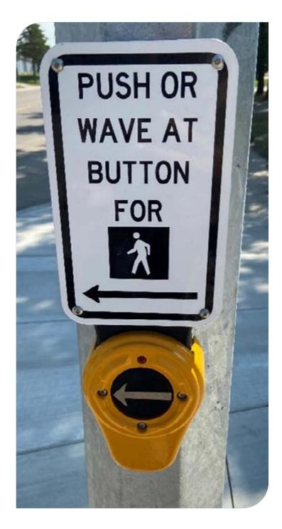
In Saskatoon, we're making crossing the streets safer for people with low vision. We now have Accessible Pedestrian Signals (APS) at 193 out of 323 signalized intersections across the city. Touchless APS are installed at 25 of these intersections. These signals use sounds to help know when it is safe to cross.
