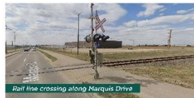
Rail line crossing along Marquis Drive
