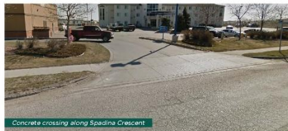
Concrete crossing along Spadina Crescent
