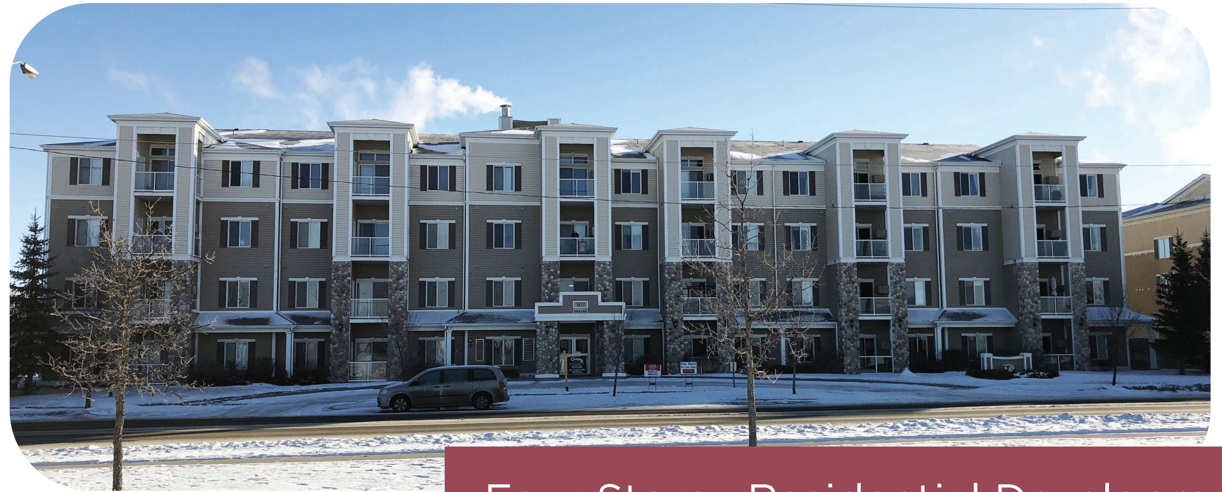
Four Storey Residential Development
