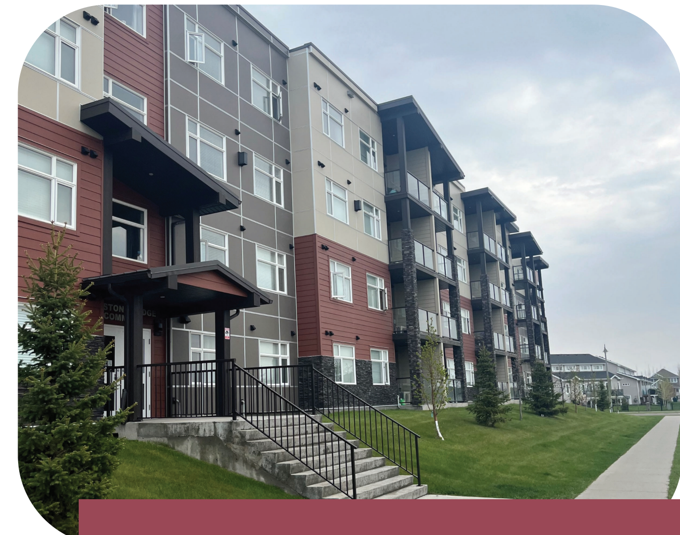
Four Storey Residential Development
