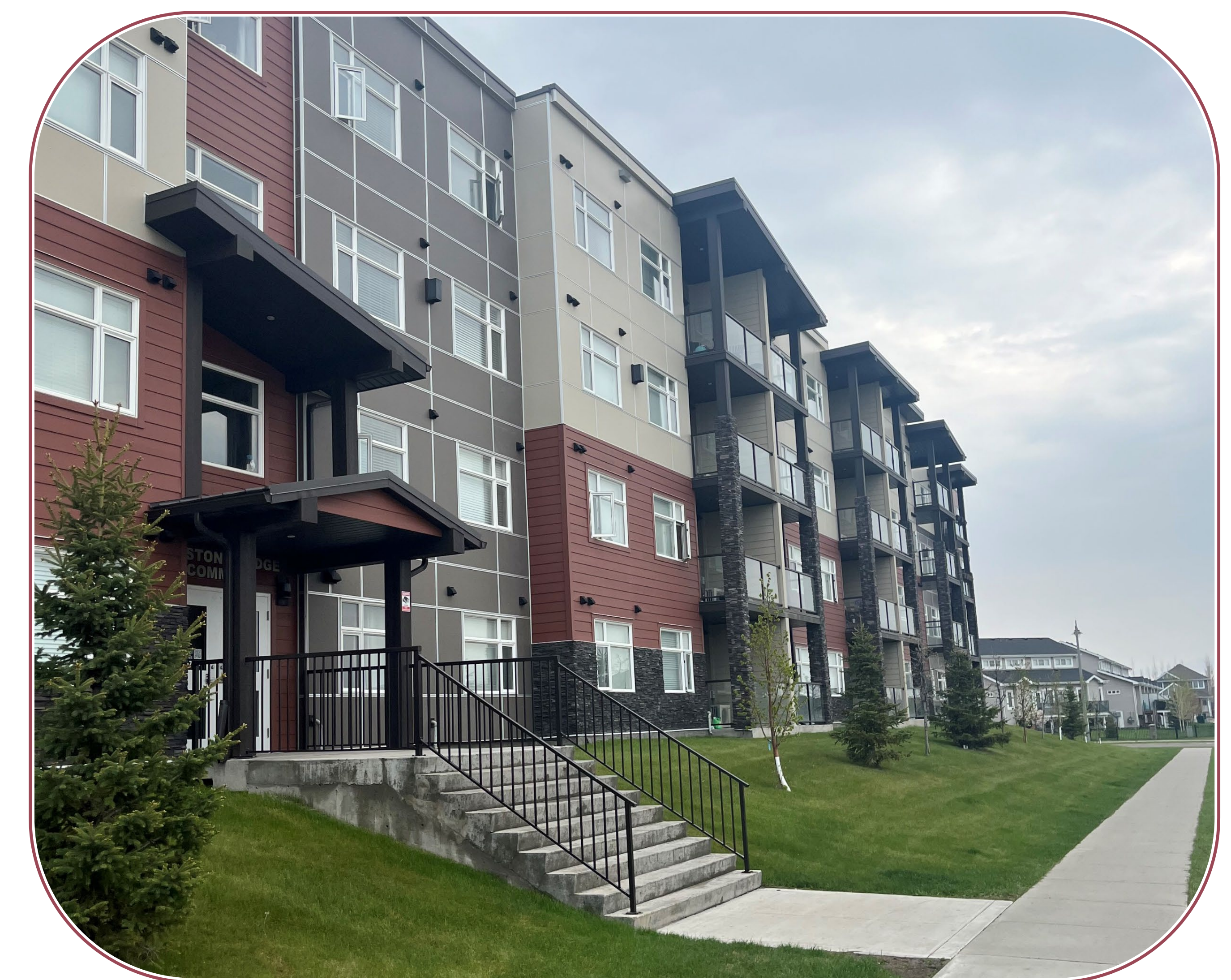
Four Storey Residential Development
