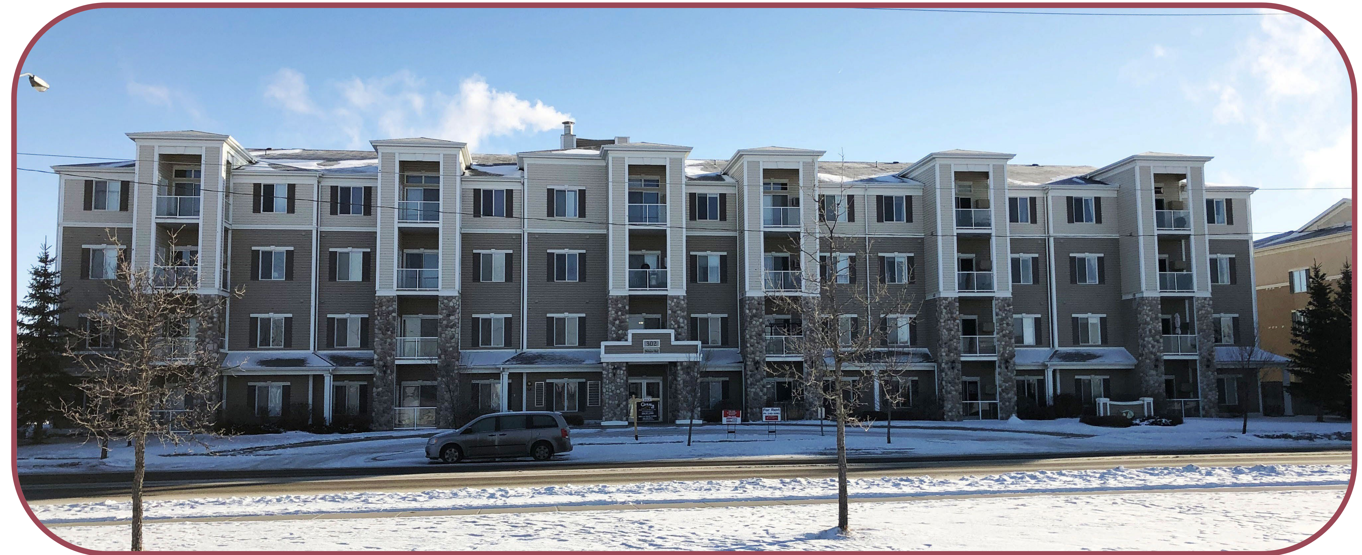
Four Storey Residential Development
