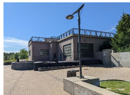
Looking west towards the A.L. Cole Pump House, a Heritage Register Property
