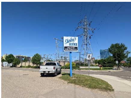
Electrical substation on Avenue C South
