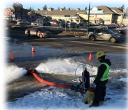
Figure 37: Fire Flow Testing
