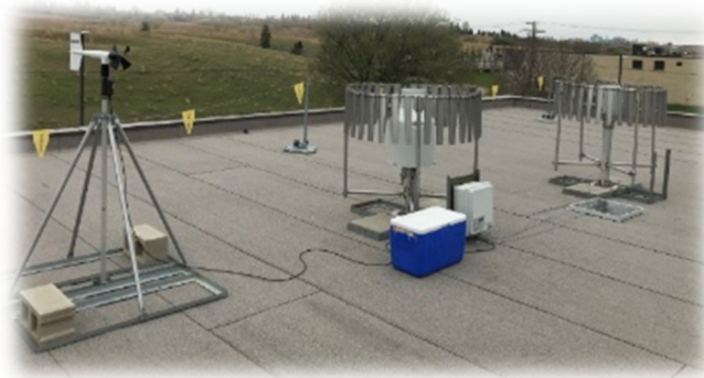
Figure 36: Photograph of Rainfall and Wind Measurement Equipment
