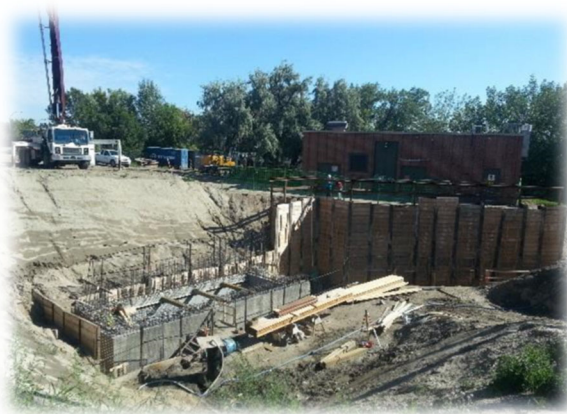
Figure 5: Photograph of Lift Station Infrastructure Construction
