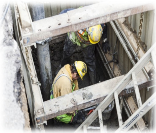
Figure 29: Photographs of Water Main Break Repair Work
