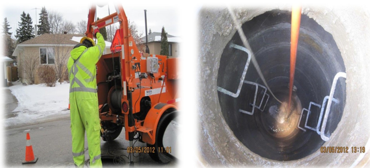
Figure 32: Photographs of Closed-Circuit Television Inspection Work
