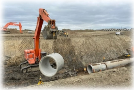
Figure 38: Brighton Storm Trunk Installation
