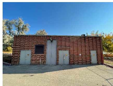
Figure 33: Spadina Lift Station
