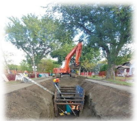
Figure 7: Photograph of Work in an Excavated Trench
