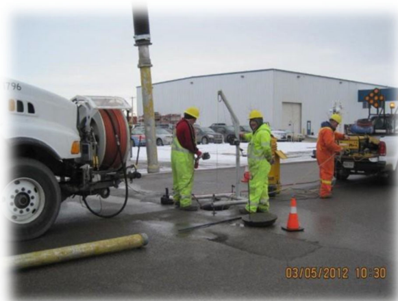
Figure 6: Photograph of Sewer Inspection Activities
