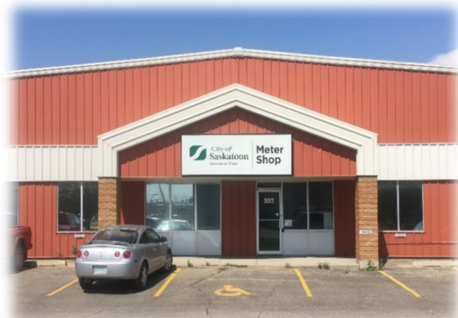
Figure 3: Photograph of the Meter Shop
