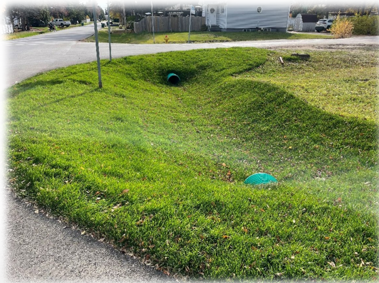
Figure 5: Completed Ditch Improvements in Montgomery Place
