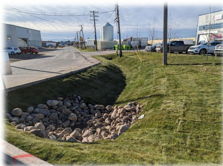
Figure 6: Completed Ditch Improvements in CN Industrial
