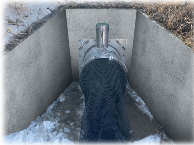
Figure 13: Image of Outfall Net
