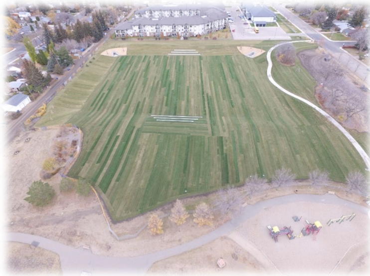
Figure 2: Churchill Park Dry Storm Pond
