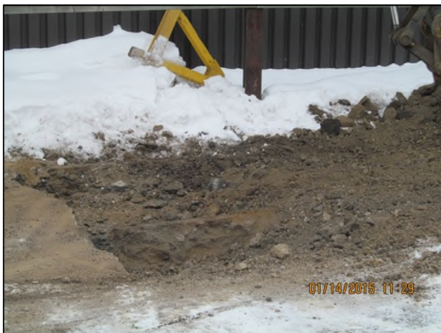
Photo 3: The excavation site, looking south.
