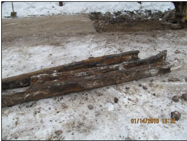
Photo 7: Historical trolley tracks removed from the excavation site.
