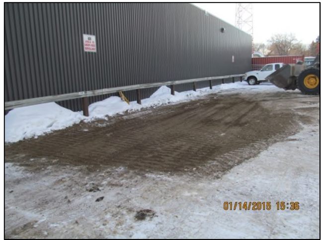
Photo 8: Backfilled excavation site, looking southwest.
