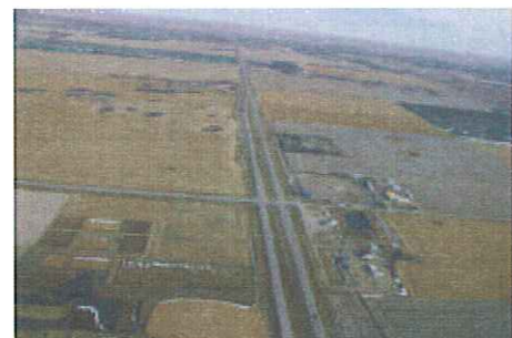
HIGHWAY 5 EAST & 41 INTERSECTION
