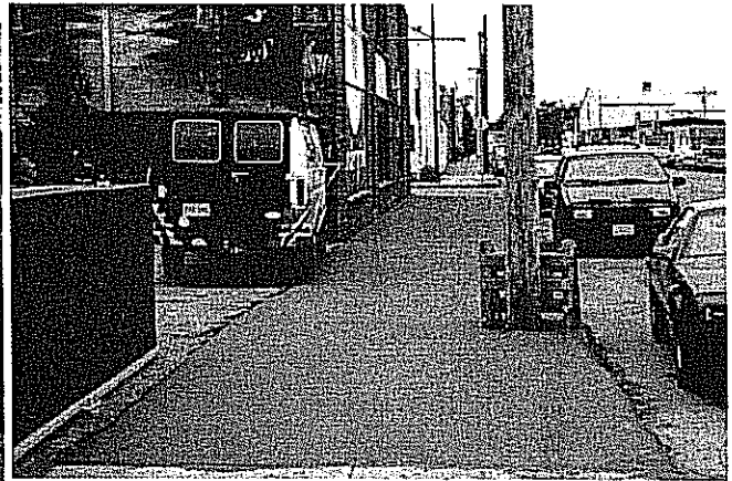
21 st Street after Sidewalk overlay - 2003
