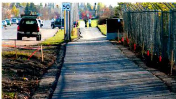
Trail construction along Lowe Road.
