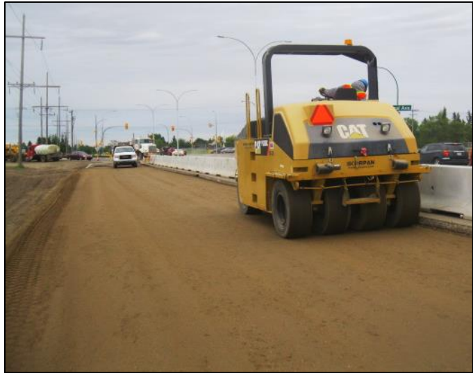
Base compaction on the added Attridge Drive lane.
