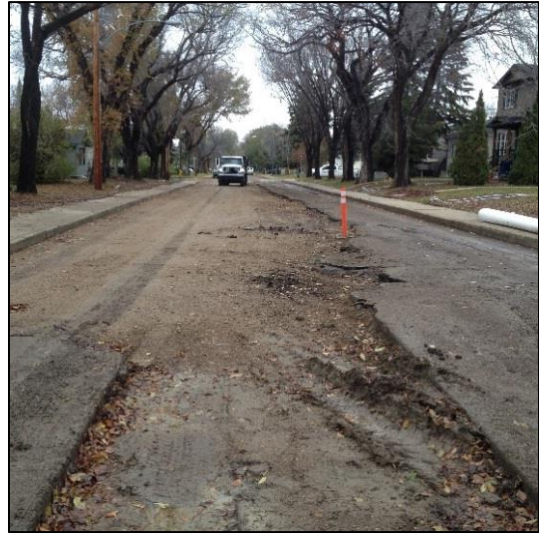
Base restoration progress over new water main.
