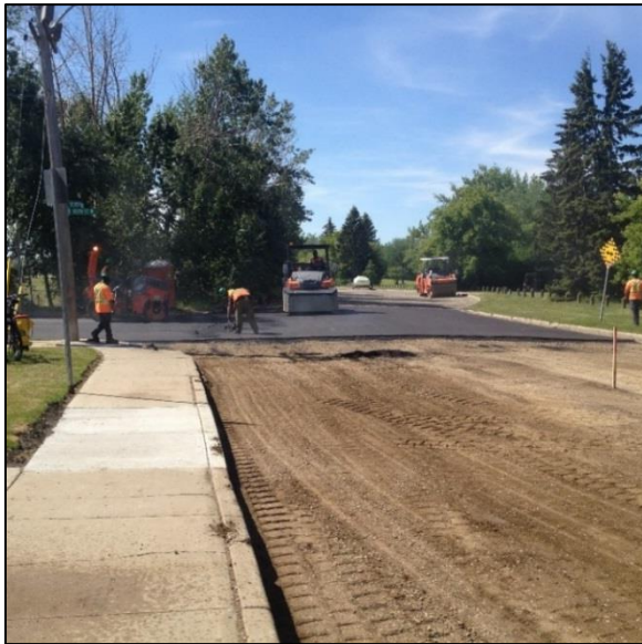
Paving over new base structure.
