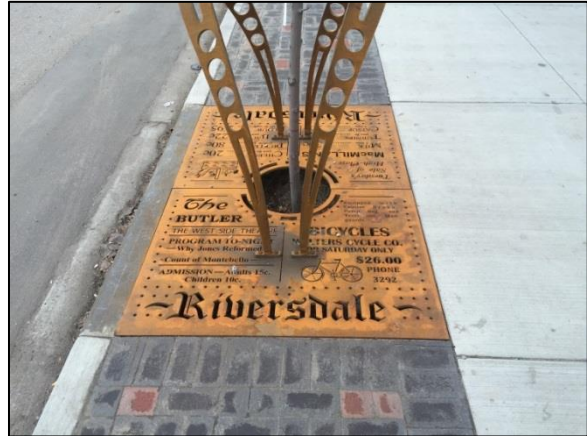
Tree gate and gutter opening for street tree.
