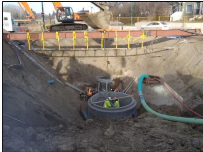
Installing sanitary chamber.
