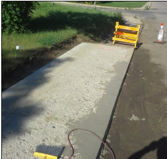
Overgrowth cutback and re-establishment of curb.
