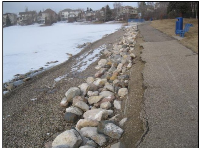
Old retaining wall and pathway.
