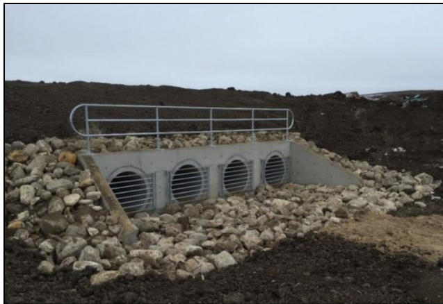
Storm sewer culvert inlets in drainage channel.
