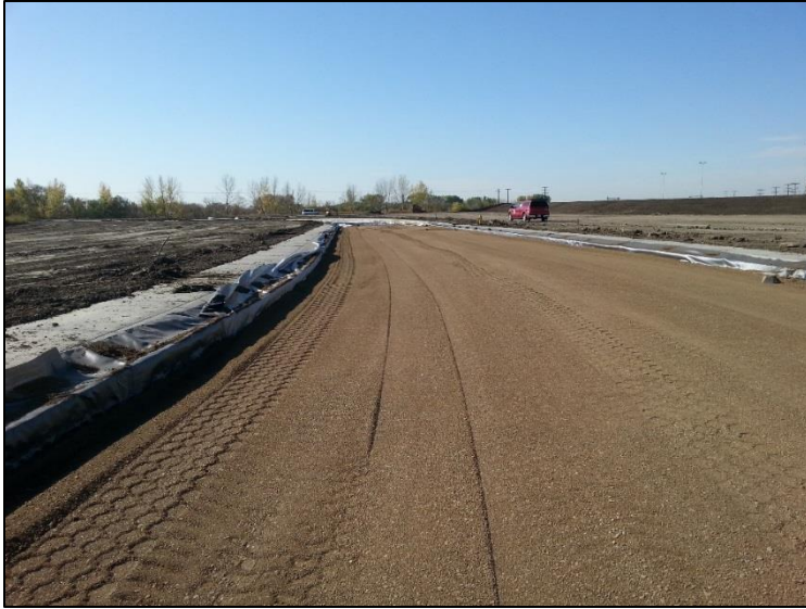
Compacting and shaping the natural fines material.
