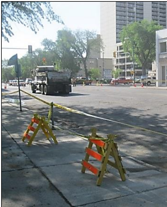
Before resurfacing 23 rd Street West.
