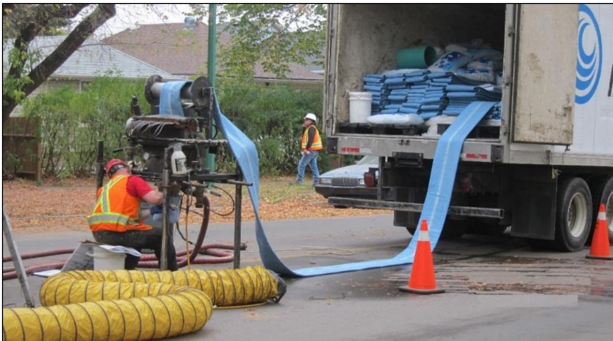
Lining sanitary sewer main.
