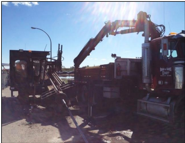
Drilling and pushing pilot rod for pipe installation.
