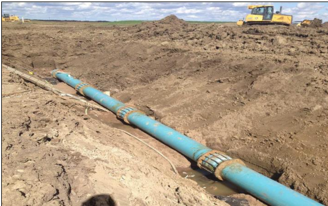
Primary water main installation with restrained joints.
