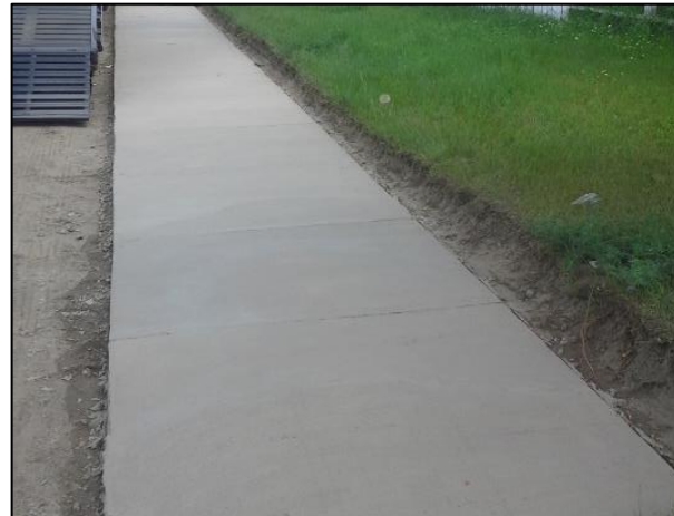
Finished MG-Krete overlay.
