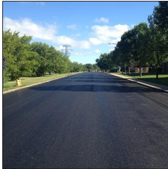
Finished asphalt surface.
