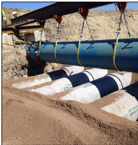
Working under existing sanitary forcemain.
