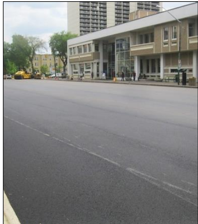
After resurfacing 23 rd Street West.
