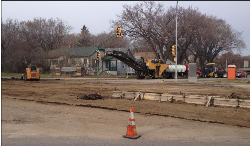
Roadway restored, awaiting paving.
