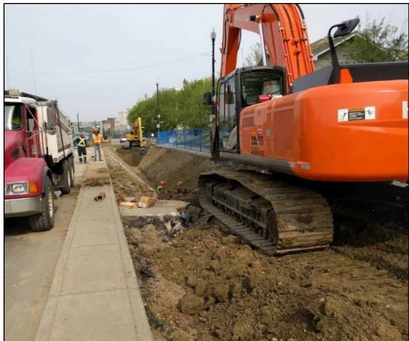
Installing water main between Broadway Bridge and 12th Street East.
