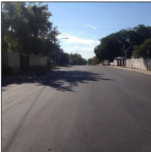
Completed base restoration over new water main.
