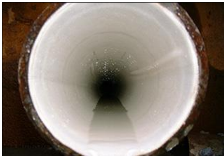
New liner installed in water main.
