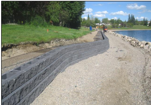
New retaining wall.
