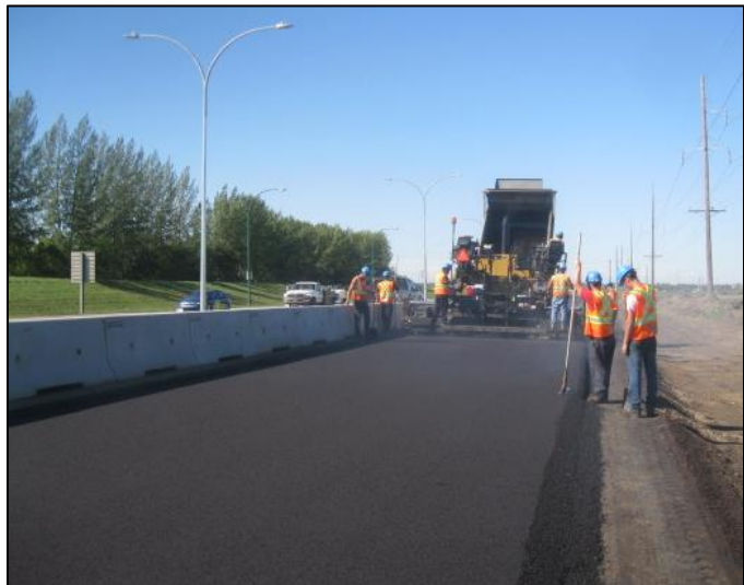
Paving bottom lift of asphalt.
