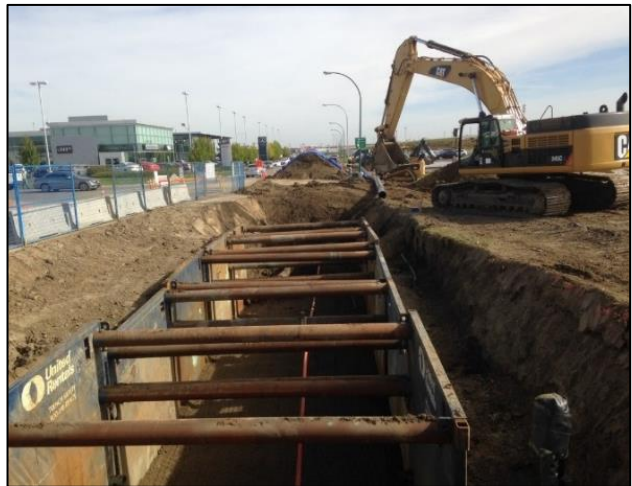
Preparing to pull pipe after reaming.
