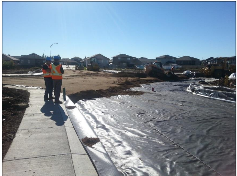
Placing natural fines material on the woven geotextile.
