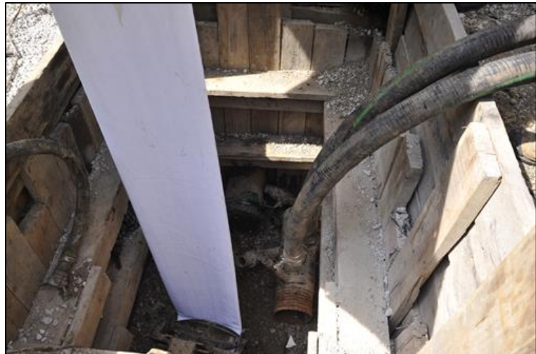
Contractor feeding liner into water main.
