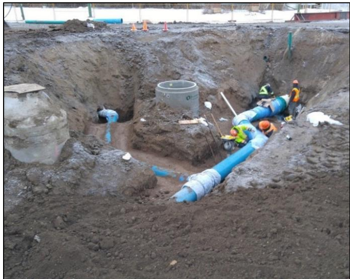
Installing sanitary main and leads.
