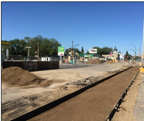
New sidewalk forms.
