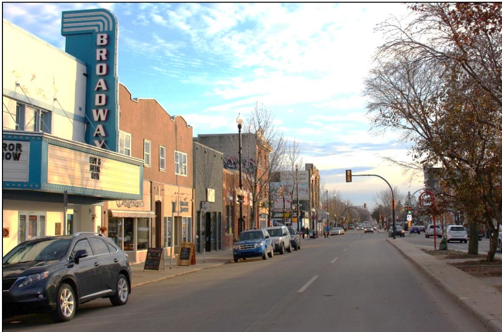
Final resurface of Broadway Avenue.
