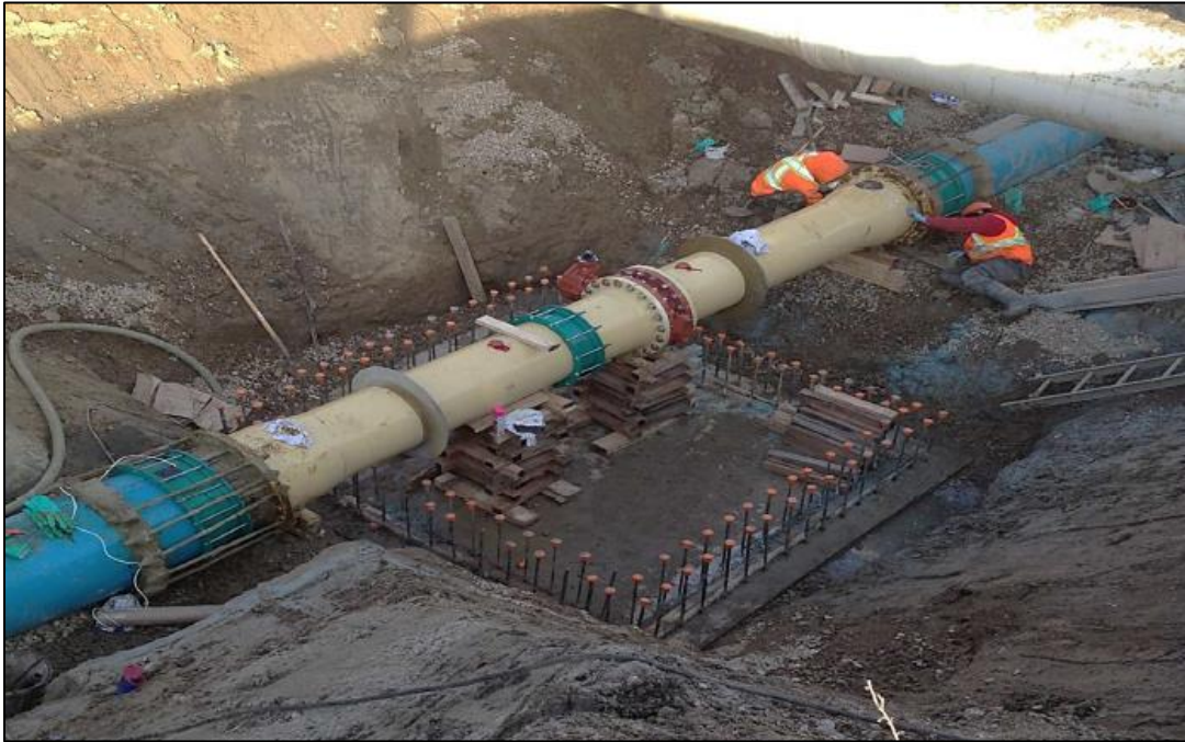
Valve chamber construction.
