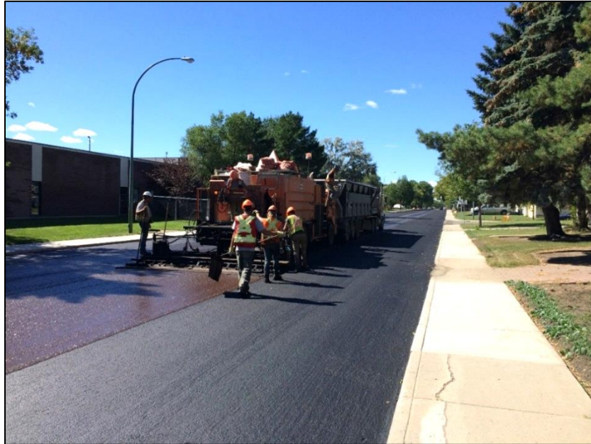
Application of micro-surfacing.
