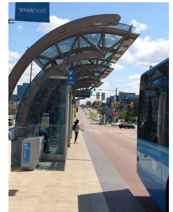
Figure 4.02 - Completed BRT Station
