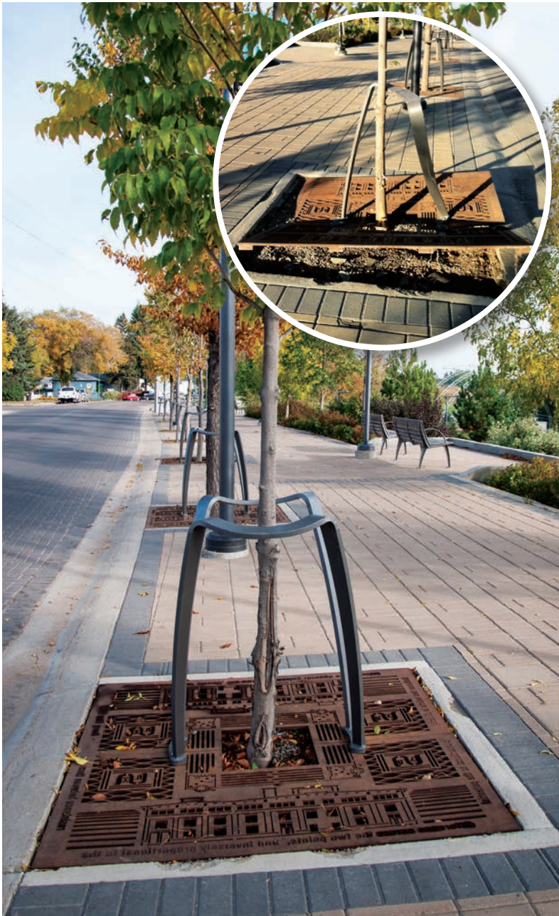
A tree grate and tree guard at River Landing were recently damaged during a motor vehicle accident. The tree grate was repositioned back into place and the tree guard was replaced, as it was damaged beyond repair.
