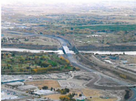
Trail has been constructed along Circle Drive South.
