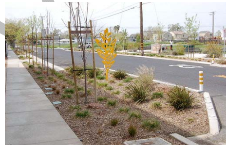
Figure 10: Stormwater bump out example
