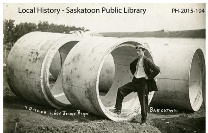
72 inch Sewer Pipe in Saskatoon, between 1912 and 1915 (Saskatoon Library, 2016)
