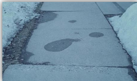
Mud Jacking or Replacement
