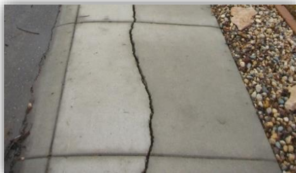
Repair - Crack Fill
