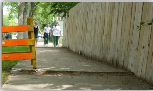
Repair – Grinding or Saw Cut
