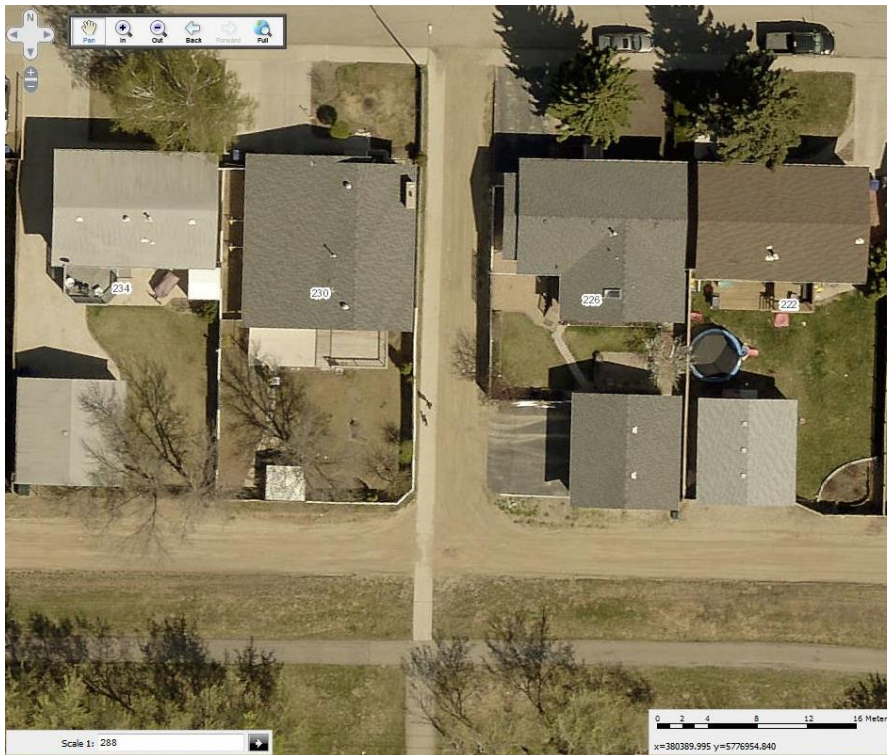
Figure 3: Dickey Crescent sidewalk in the back lane.
