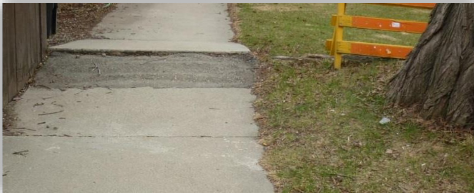
Tree Root – Replacement
