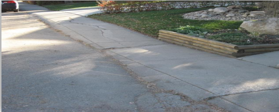
Utility Settlement – Mud Jack or Replacement
