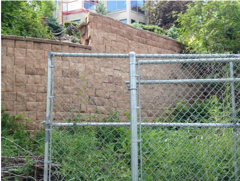
Photo C.9. Retaining Wall in Backyard of 237-239 11th St. E. (June 21, 2012)
