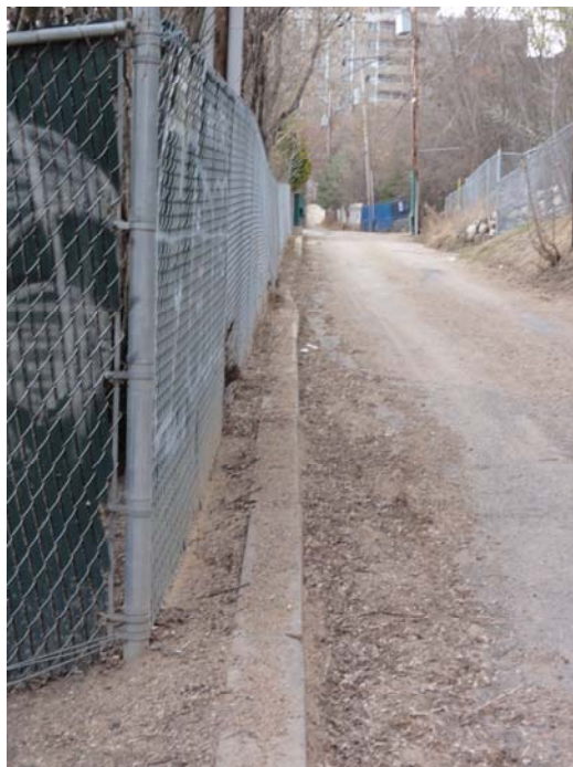
Photo C.3. Looking East at Deflection of Curb and Fence Line along Cherry Lane (April 26, 2012)
