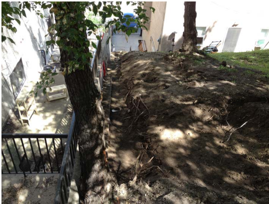
Photo C.28. Looking North at Partially Filled Trench (July 17, 2013)
