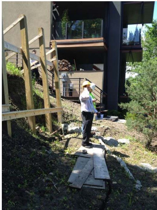
Photo C.11. Cracking along Headscarp of East Failure (June 21, 2012)
