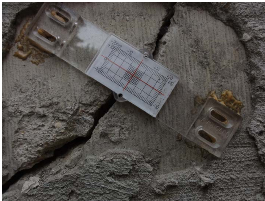
Photo F.4: Crack Meter Located on the East Face of the Retaining Wall Between 230 & 306 Sask. Cres. E. (CM2) (Sept 18, 2013)
