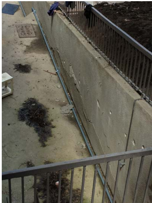
Photo C.25. Looking Northeast at Concrete Retaining Wall between 230 & 306 Sask. Cres. E. (July 7, 2013)
