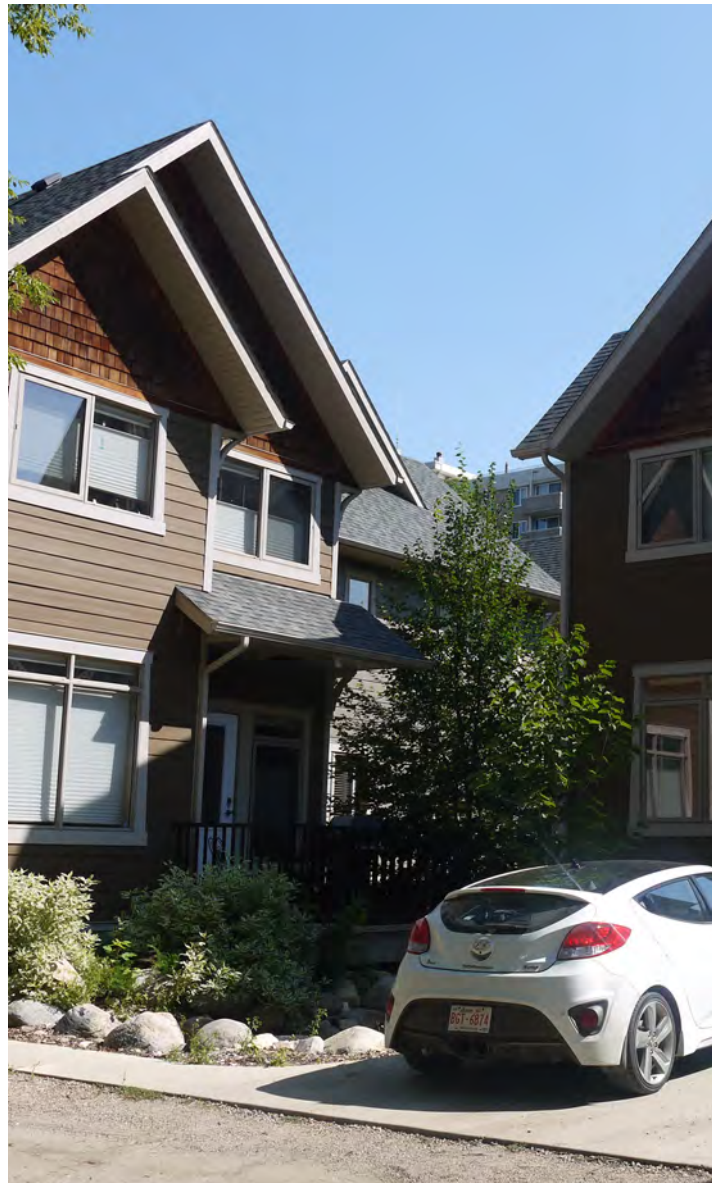
Buildings should not have blank facades. Flanking facades should have a design and material standard equal to the primary facade.
