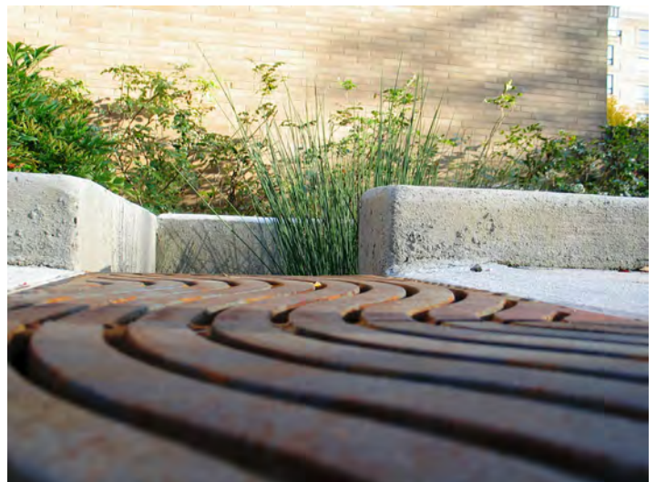
Well-drained snow storage areas should be provided on site in locations that enable melting snow to enter a filtration feature.
