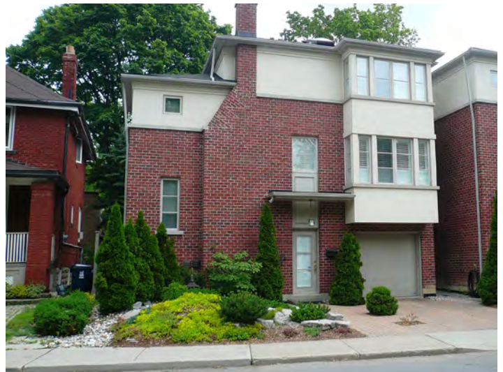
3 metres of the minimum 6 metre front yard setback should be free of encroachments and dedicated to front yard landscaping.
