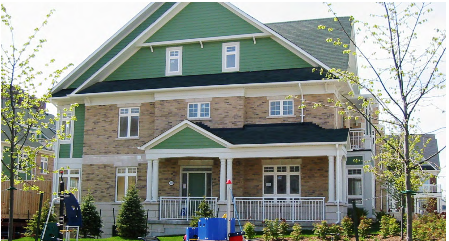
On a corner lot condition, dual frontage should be incorporated through the use of wrap-around porches, sun rooms, bay windows, and secondary side yard entrances.
