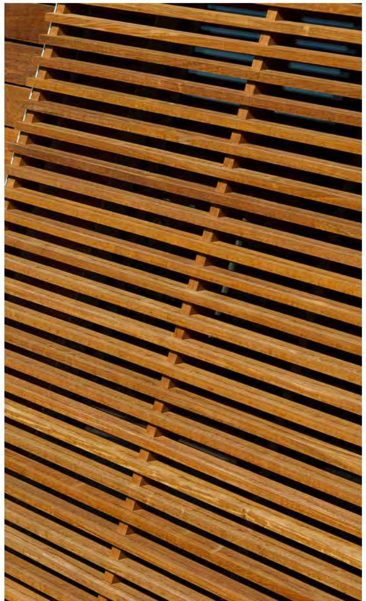
Example of a screening element for garbage and recycling storage within a garden and garage suites.
