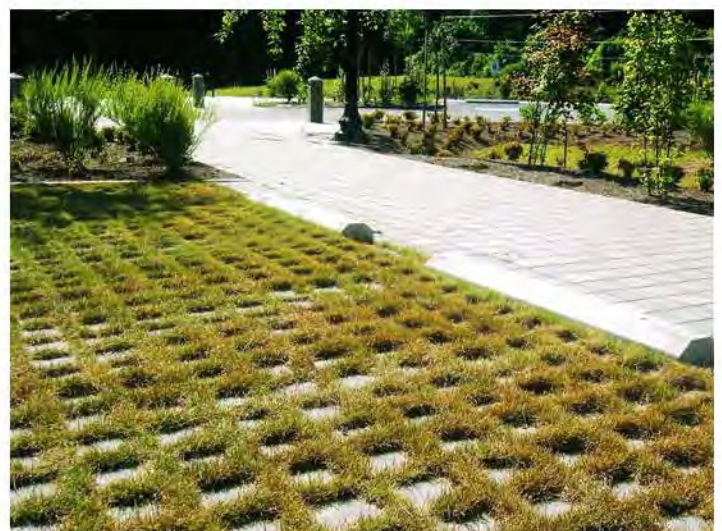
Porous pavement, and landscaped areas with adequate size and soil conditions, should be maximized to capture roof drainage and increase the total amount of absorbed run-off infiltration.
