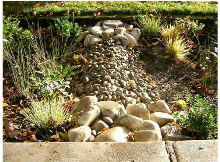
Landscape design should incorporate strategies to increase the total amount of absorbed run-off infiltration.
