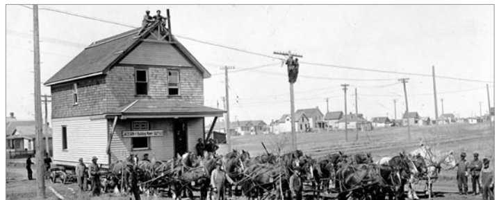
A house being moved east along 33rd Street near Avenue A by “Jackson the Building Movers”, c. 1916 (Saskatoon Public Library Local History Room LH-4774)
