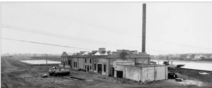
Water treatment plant at 11th Street West and Avenue H, 1914 (Saskatoon Public Library Local History Room LH-1824)
