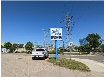
Electrical substation on Avenue C South
