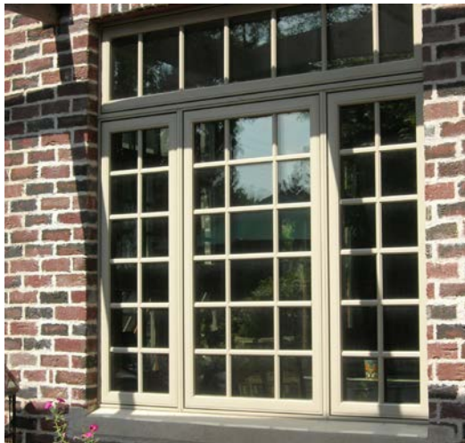
Brick Exterior with Tall Narrow Windows (2014)
