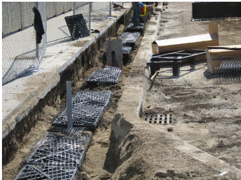
Figure 22: 3rd Avenue Saskatoon in 2010, Silva Cell installation
