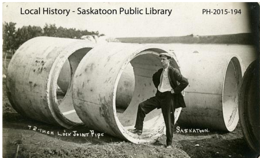
Figure 1: 72 inch Sewer Pipe in Saskatoon, between 1912 and 1915 (Saskatoon Library, 2016)
