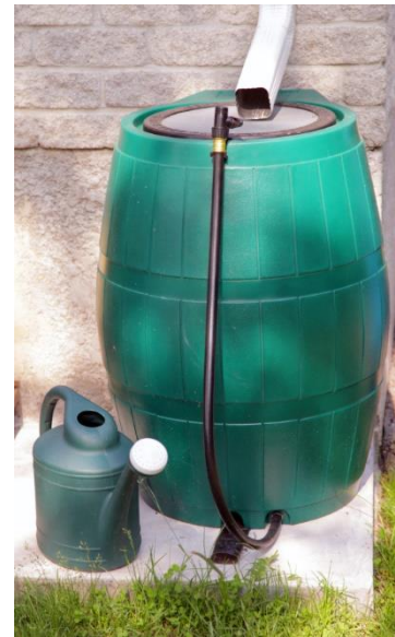
Figure 26: Residential rain barrel
