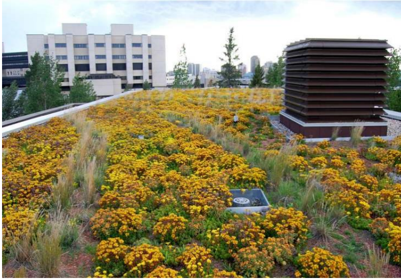
Figure 17: College of Law Addition Green Roof, Saskatoon
