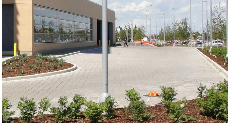
Figure 20: Permeable Pavement Walkway in Calgary (photo courtesy Expocrete)
