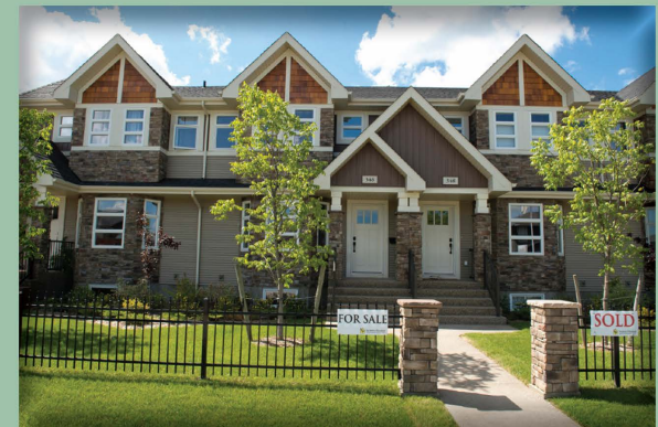
Above: Each of the above images demonstrates a minimum of two exterior cladding materials with sensitively designed proportions.
