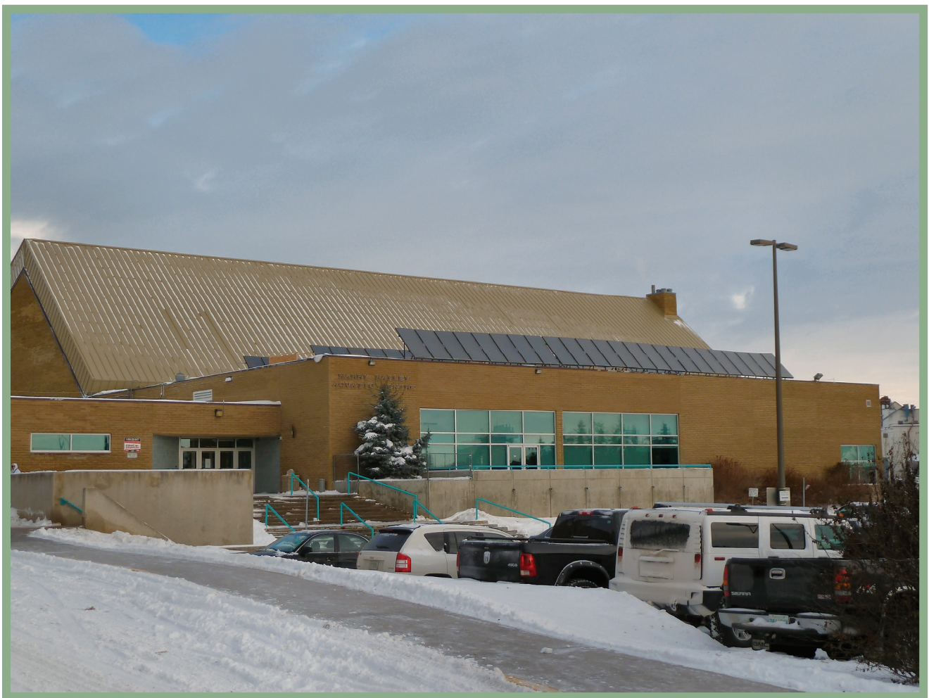
New Solar Panels Installed at Harry Bailey Aquatic Centre
