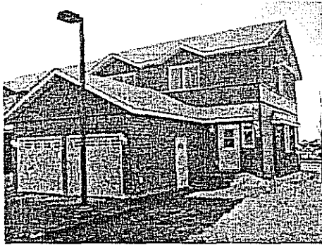
Modular Built townhouses, sold through the Mortgage Flexibilities Support Program, 715 Hart Rd
