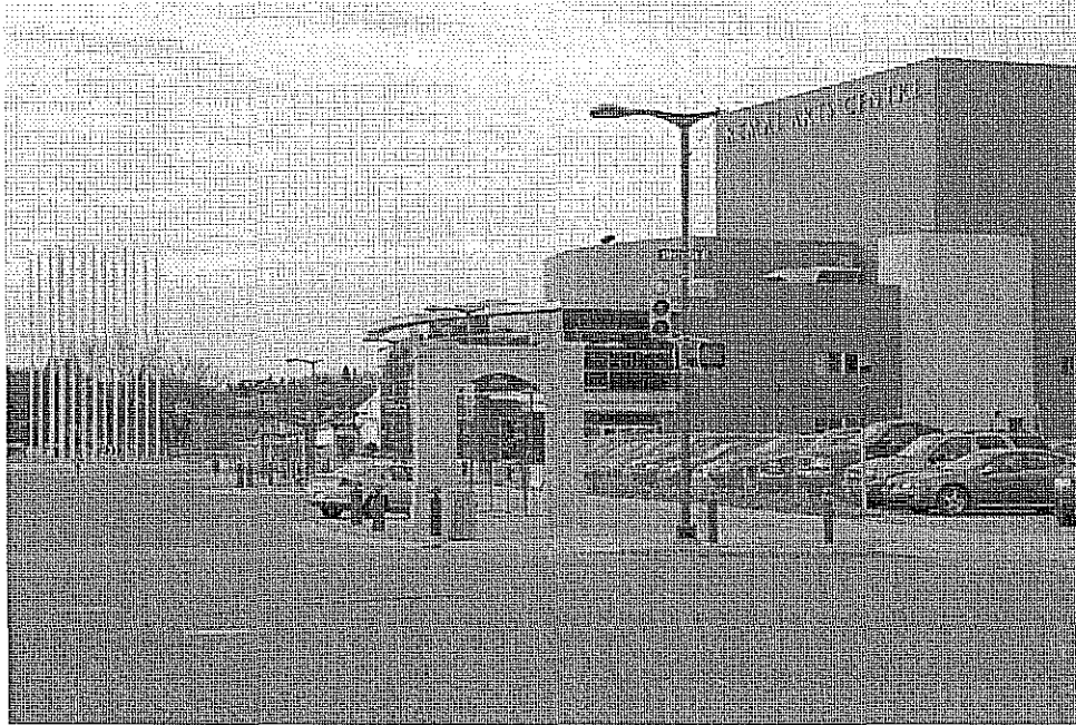
View South on 2 nd Avenue
