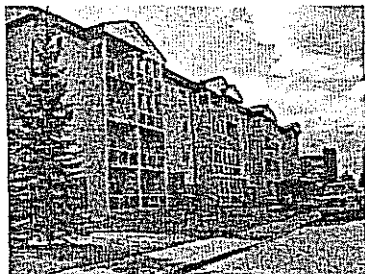
Bethany Manor, 110 La Ronge Road, featuring geo-thermal heating.
