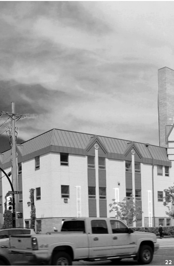
22 existing site condition looking north from 25th St. E.
