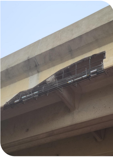
108th Street Overpass Emergency Repairs
