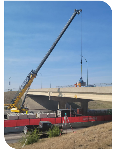
108th Street Overpass Emergency Repairs
