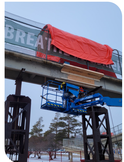
Emergency Repairs to Campus Pedestrian Bridge
