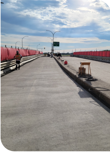
Attridge Drive Overpass Rehabilitation
