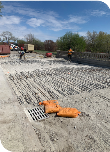
Spadina Crescent Bridge - Deck Demolition
