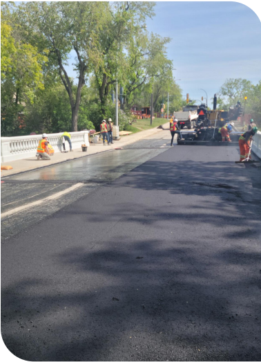
Spadina Crescent Bridge - Resurfacing
