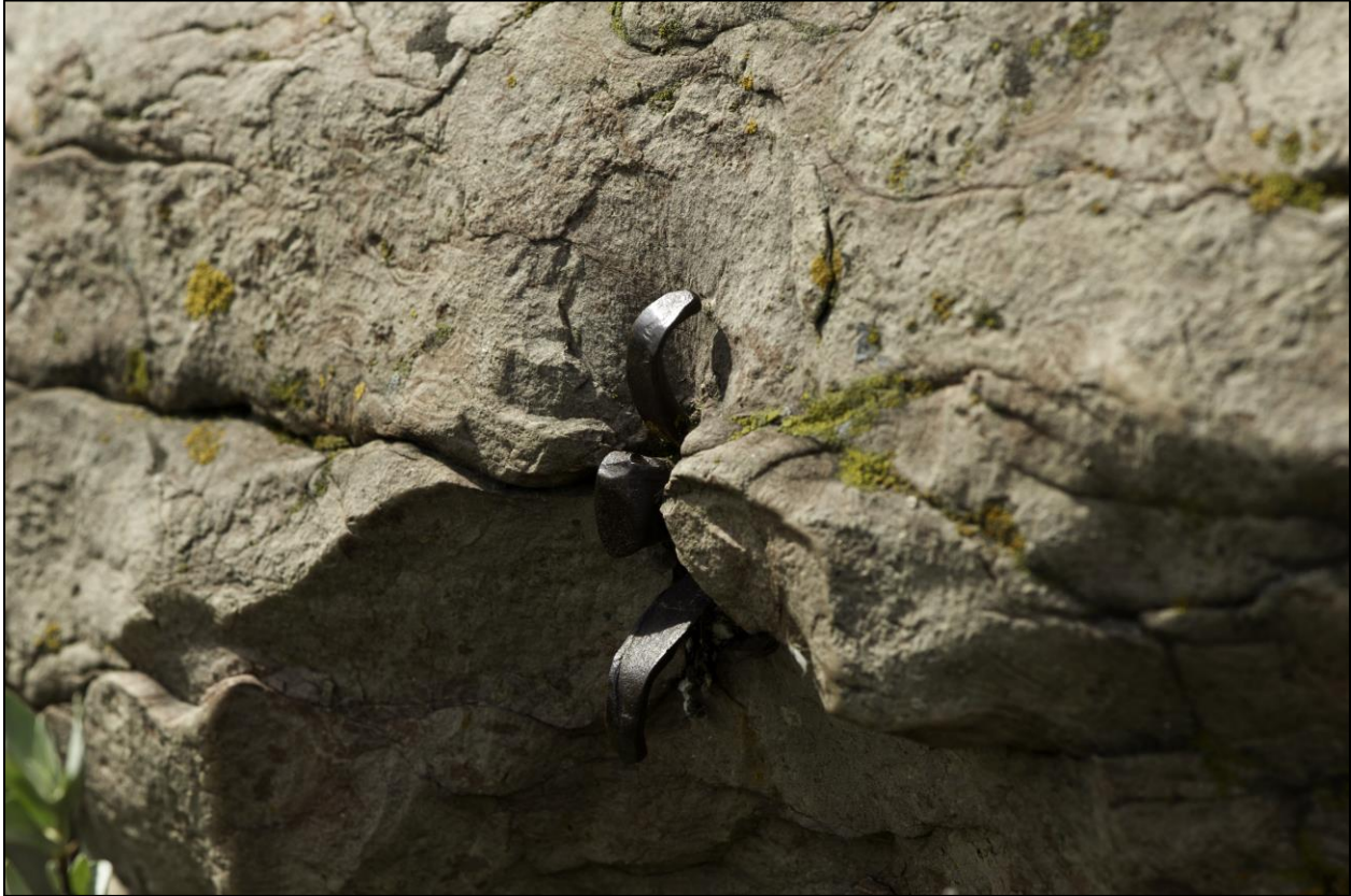
Figure 23 Pinned Rock (DAFT Media, 2011)
