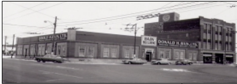
Photo taken from the corner of Idylwyld Drive and 23 rd Avenue. The Fairbanks Morse Warehouse is seen on the right. 26
