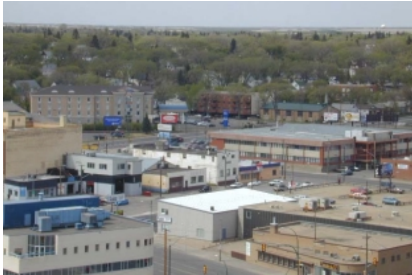
New and old structures comprise the Warehouse District
