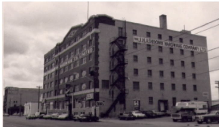
Ashdown Warehouse: Destroyed by fire in 1995 27
