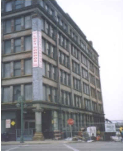
The exterior of a loft conversion in progress, Downtown Milwaukee
