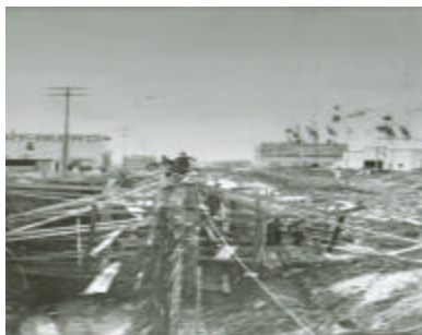
Construction of the subway. 10
