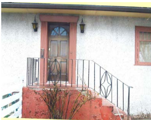
Side Entrance Stairs (2014)
