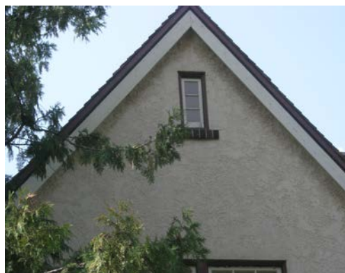
Steeply Pitched Roof (2014)
