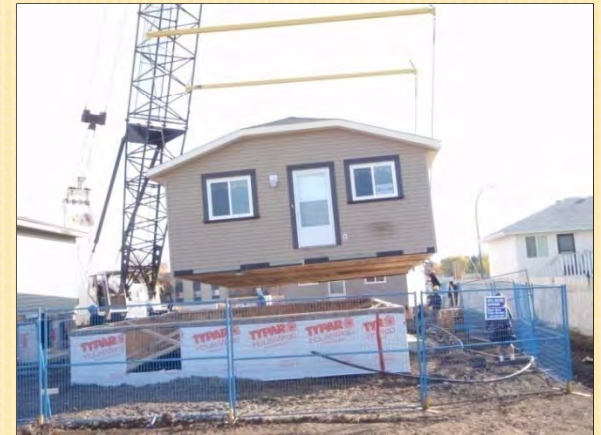
Borden Crescent Affordable Housing
