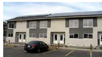
Solar Thermal and Electric Panels on Affordable Townhouses, Pleasant Hill Village
