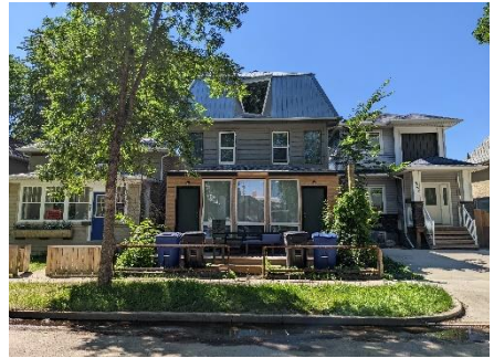
Multi-unit conversion of Riversdale character home
