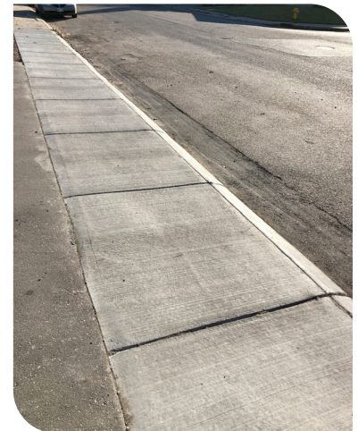
Wollaston Crescent: after
