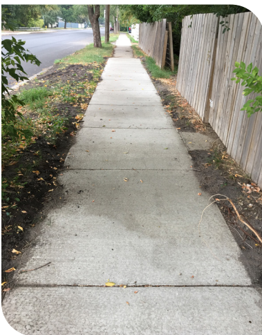
111 th Street West: after
