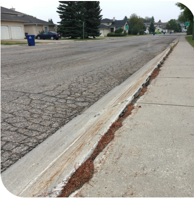
Kenderdine Road: before
