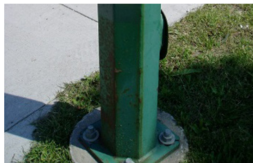
Street Light Pole in Good Condition
