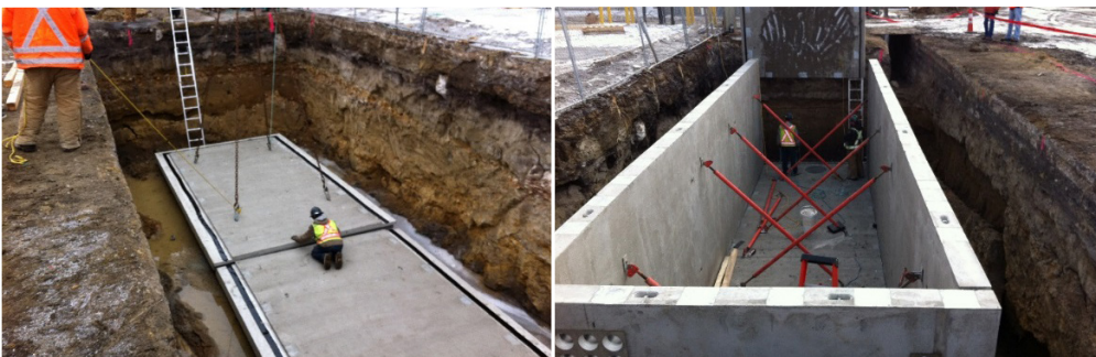
Network Vault under Construction – Floor and Walls
