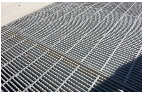
Network Vault Grate in Good Condition
