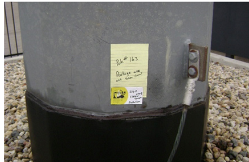
Transmission Tower Base in Good Condition
