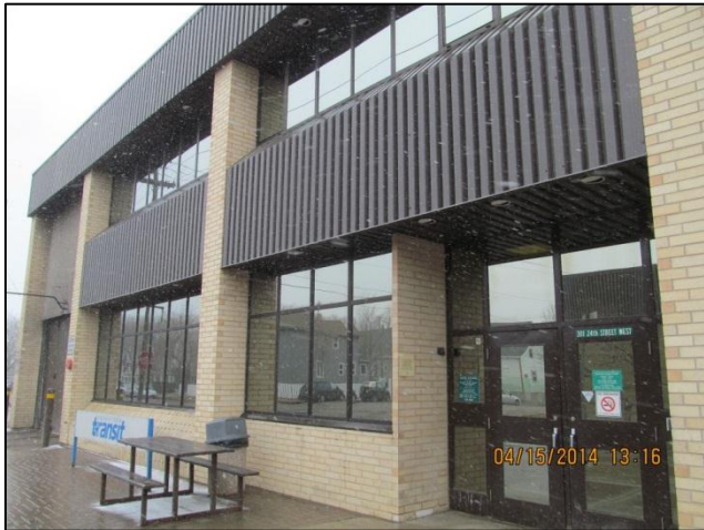
Photo 1: Main entrance of 301 24 th Street W looking southeast.
