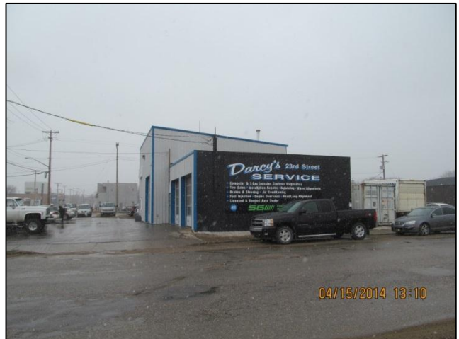
Photo 48: Darcy's 23 rd Street Service located at 304 23 rd Street W, looking west.
