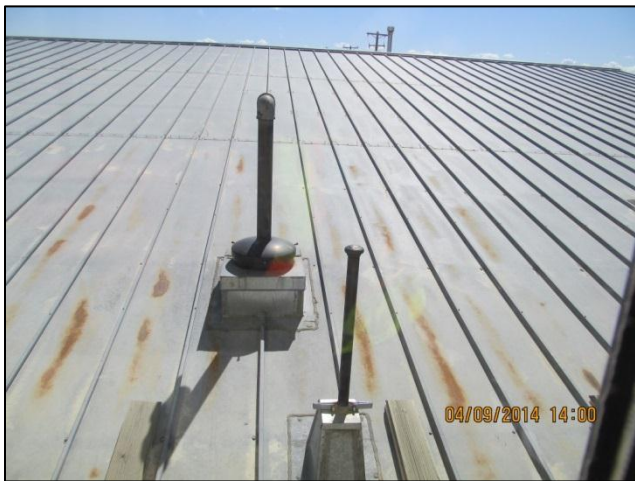
Photo 9: Vent lines spotted from 2 nd floor window, 301 24 th Street W. Vent lines are related to the back-up generator in the bus storage barn.
