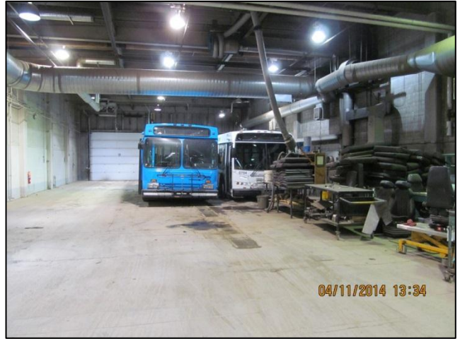
Photo 38: Shop B at 321 Ave C N looking west. Note the bus interior washing/repair station and surficial staining.
