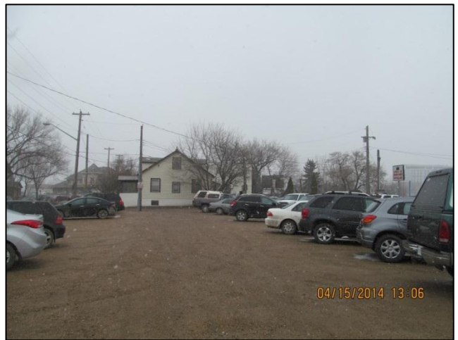
Photo 40: Transit staff parking on 230, 232, and 240 Ave C N looking east. Note the pole mounted transformer.
