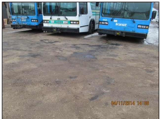
Photo 18: The storage yard in the northwest portion of 321 Ave C N. Note the hydrocarbon staining.
