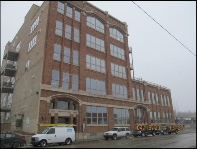
Photo 50: Residential condominiums located at 211 Ave D N looking northwest.
