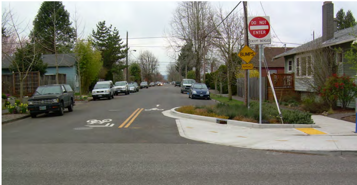
An example of a directional closure. The curb blocks one lane of traffic from proceeding through the intersection.
