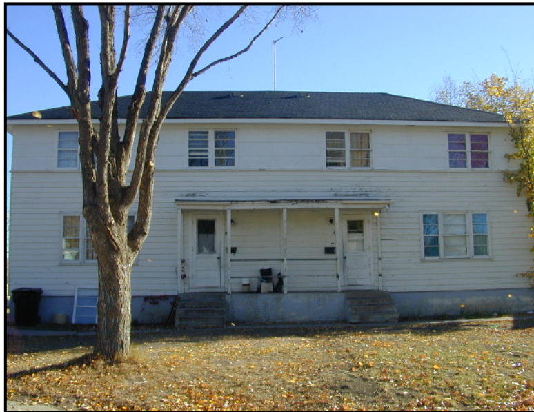
McNab Park Multiple Unit Dwelling
