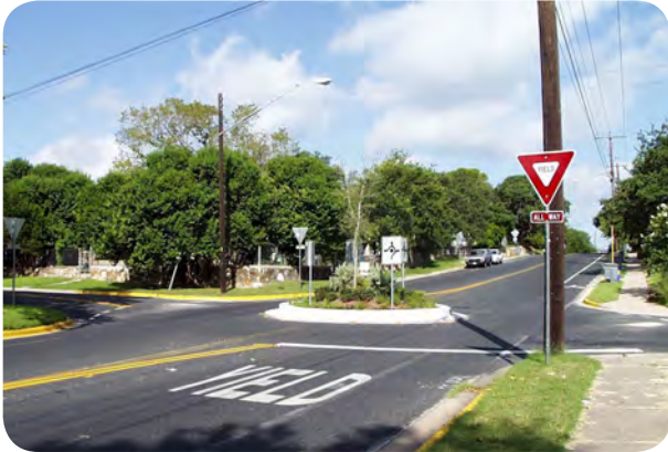
Traffic calming measures: Roundabouts.
