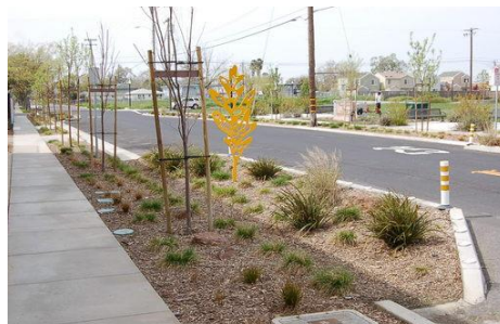
Figure 10: Stormwater bump out example
