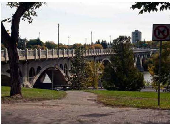
Victoria Street Bridge from east bank, Saskatoon, SK, Source: Urban Systems; University Drive Bridge from west bank, Saskatoon, SK, Source: Urban Systems
