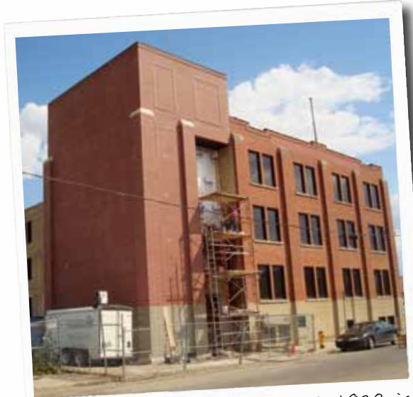
The Arthur Cook building, built in 1928, is being completely renovated.
