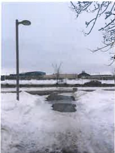
Figure 14: Walkway Lighting Concerns
