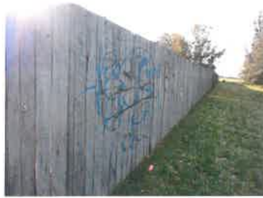
Figure 8: Further Evidence of Graffiti Vandalism
