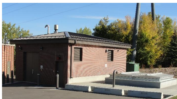
Spadina Lift Station
