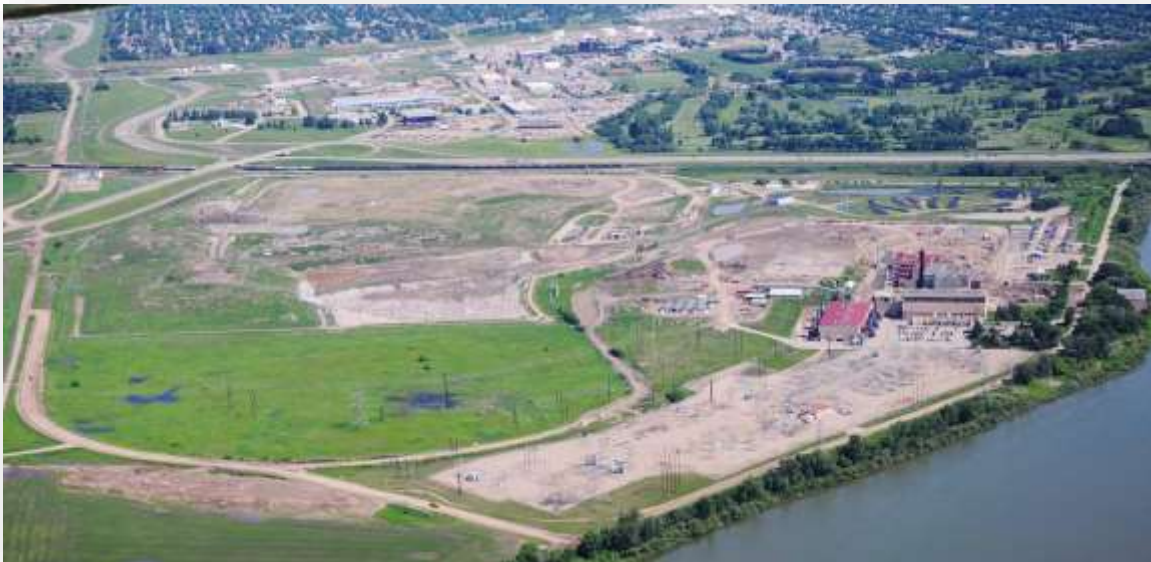
Saskatoon Regional Waste Management Facility
