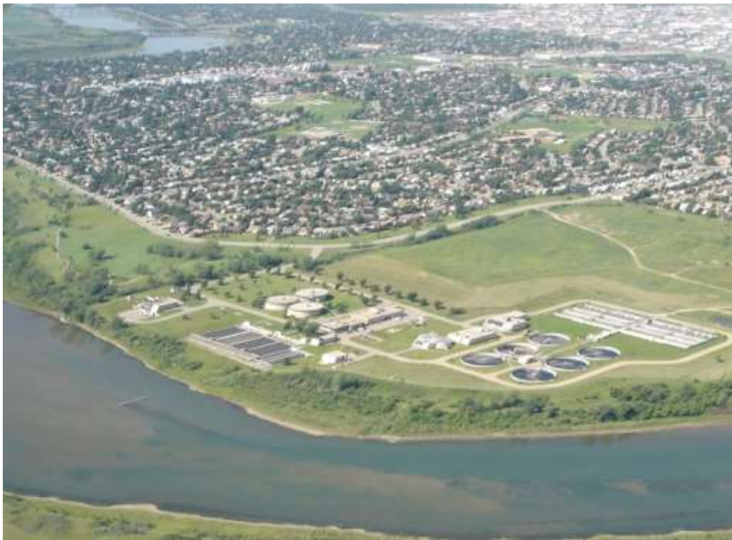
Wastewater Treatment Plant
