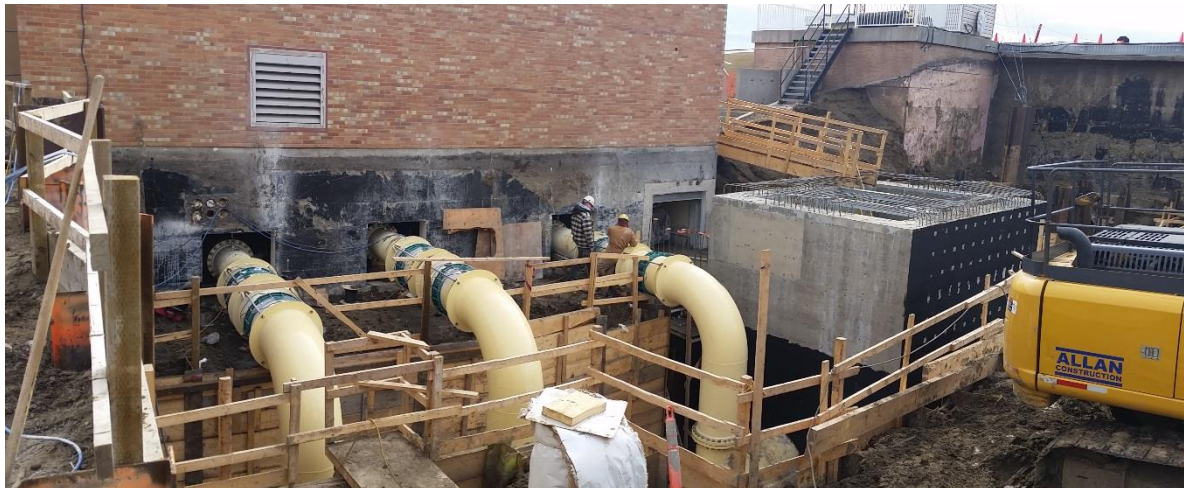
Construction on Acadia Drive Reservoir and Pumphouse
