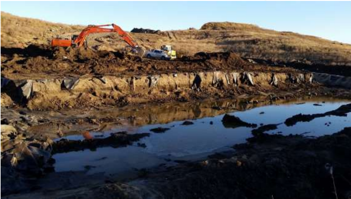
Lead Cell Excavation
