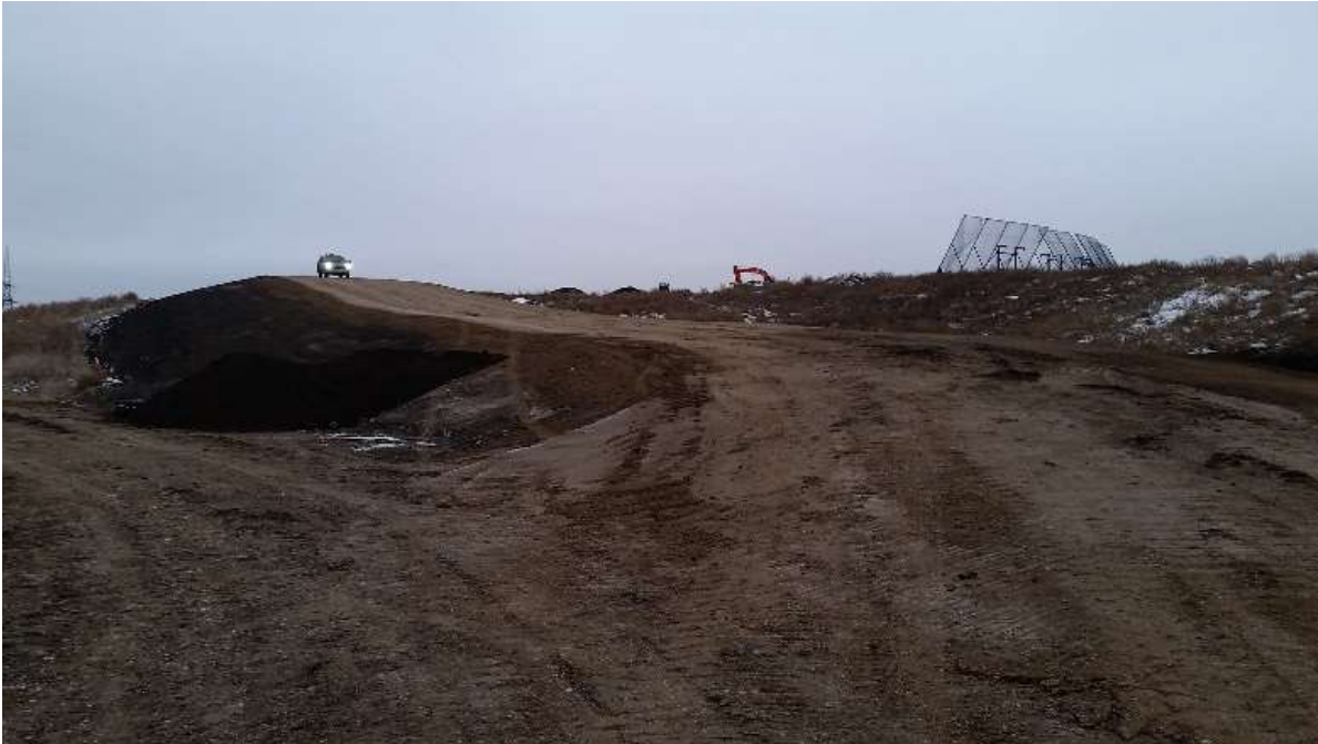
New Haul Road
