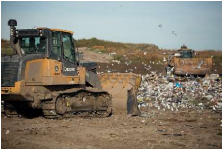
Saskatoon landfill operations.
