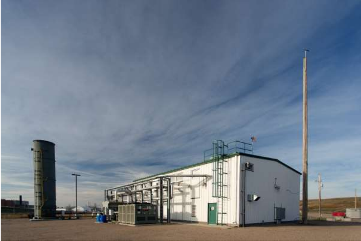
Landfill gas facility
