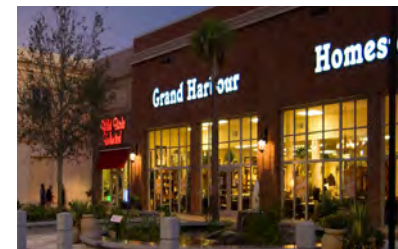
A good example of a consistent fenestration pattern
