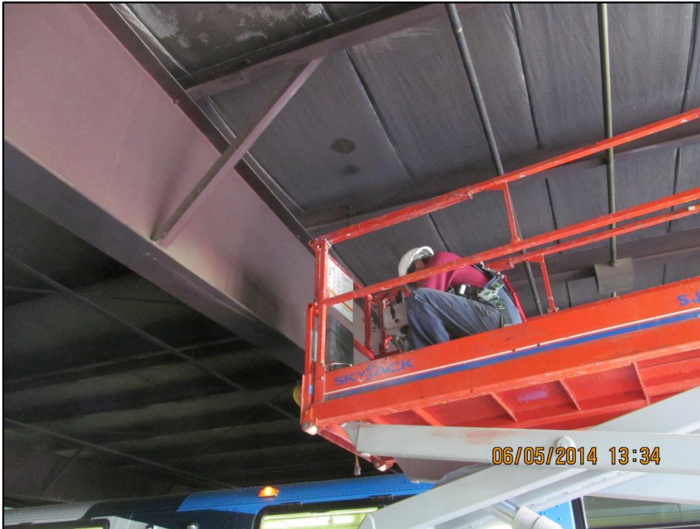
Photograph #13: Diesel particulate sampling, bus storage barn located at 301 24 th Street West.
