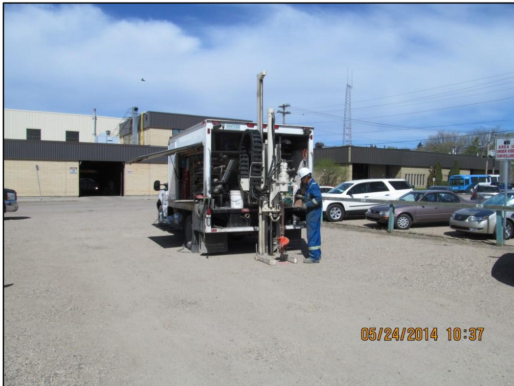
Photograph #10: Advancing borehole 14-41 at 240 Avenue C North, looking northwest.
