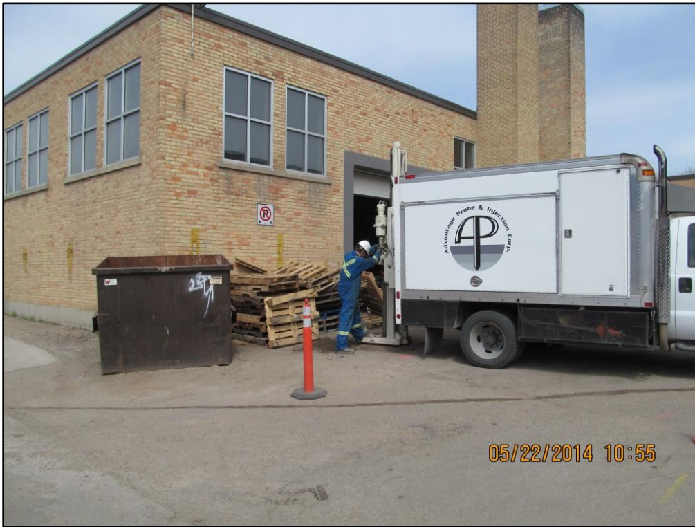
Photograph #7: Advancing borehole 14-24 in the loading area located at 321 Avenue C North.
