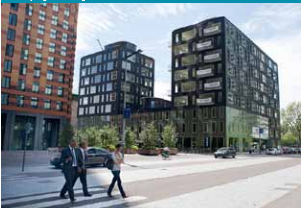
6.48 Django Building - Amsterdam
