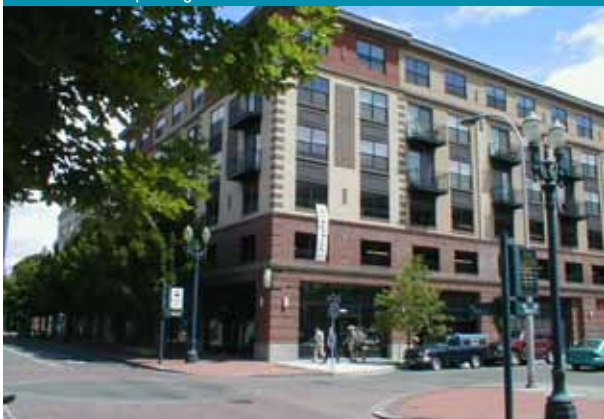
6.51 Structured parking above retail
