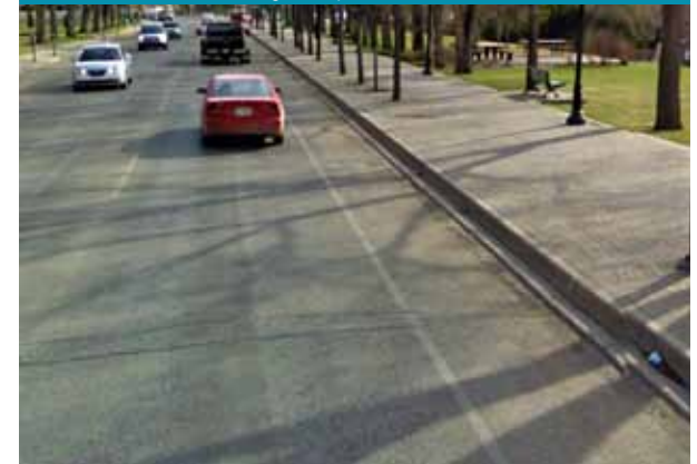
4.54 Faint Bike Lane Markings on Spadina Crescent
