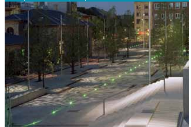
6.67 Lighted bike lane, Copenhagen
