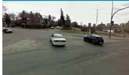
4.19 Poor markings at University & Saskatchewan Cr.
