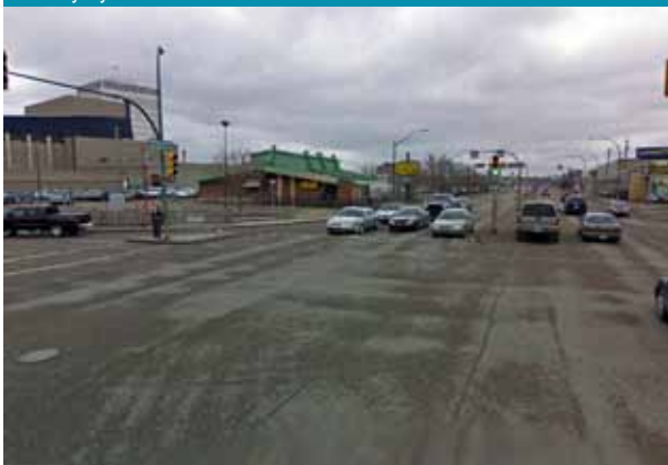
4.55 Idylwyld Drive and 22nd St.
