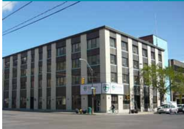
3.4 Edwards School of Business: first downtown university facility
