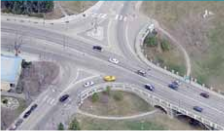
4.14 Wide intersection & underpass (Spadina @ Bridge)
