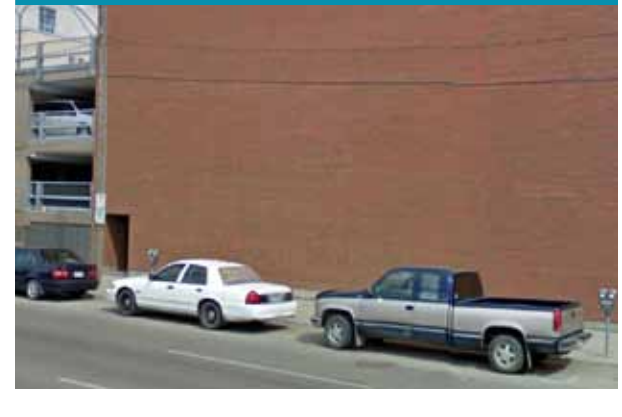
4.42 Blank wall on 1st Ave.
