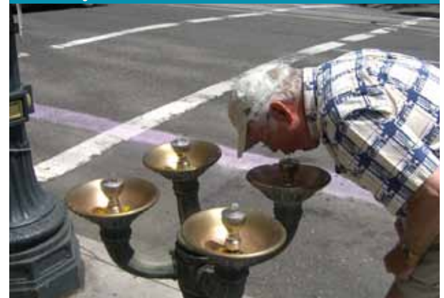
6.81 Drinking water fountains, Portland
