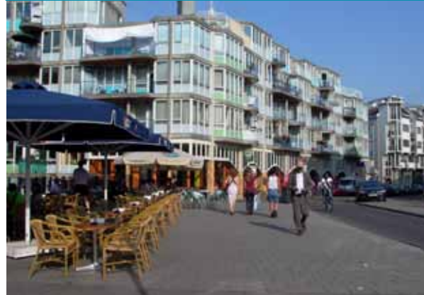
6.15 Live/work studios, Amsterdam
