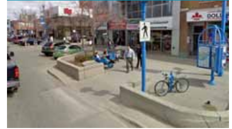
4.17 Narrowed mid-block crosswalk on 2nd Ave.
