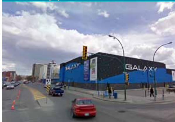
4.41 Over-scaled signage at 20th St. and 1st Ave.
