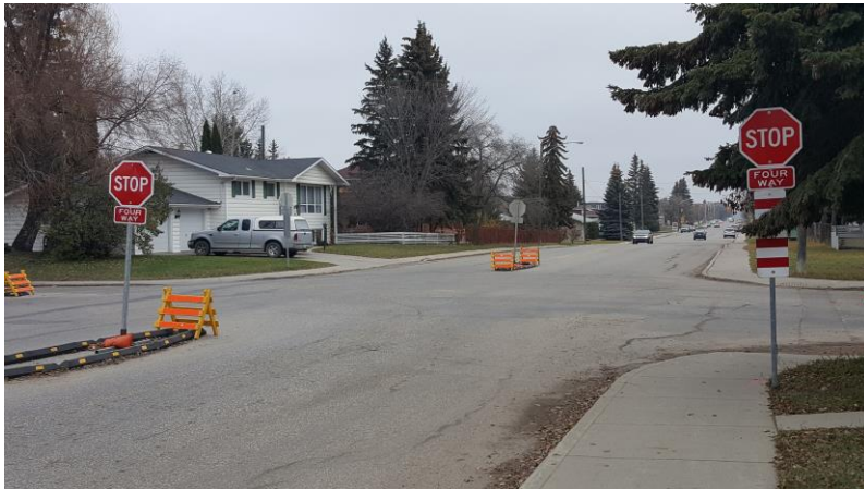
New 4-way Stop installed at Witney Avenue and 20 th Street intersection with temporary medians that will be considered for permanent installation
