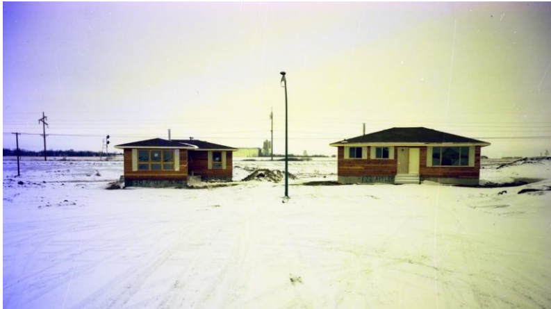
530 and 526 Appleby Place in February 1977, under construction (credit: Photograph CP-7393-B by Creative Professional Photographers courtesy Saskatoon Public Library – Local History Room)
