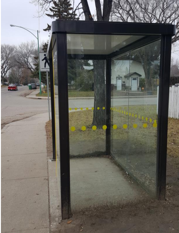
Bus shelter on Avenue W at 18 th Street
